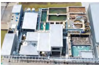
Wastewater recycling plant (MMTh)
