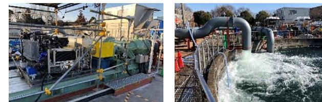
"DELICA D:5" engines driving drainage pumps
