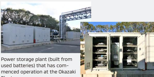
Power storage plant (built from used batteries) that has commenced operation at the Okazaki Plant
