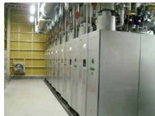
Compact through-flow boilers
